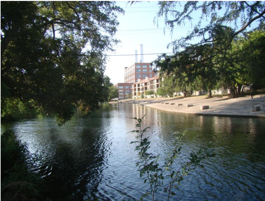
Southeast view of mill race canal towards the Landmark (LCRA) Building.
