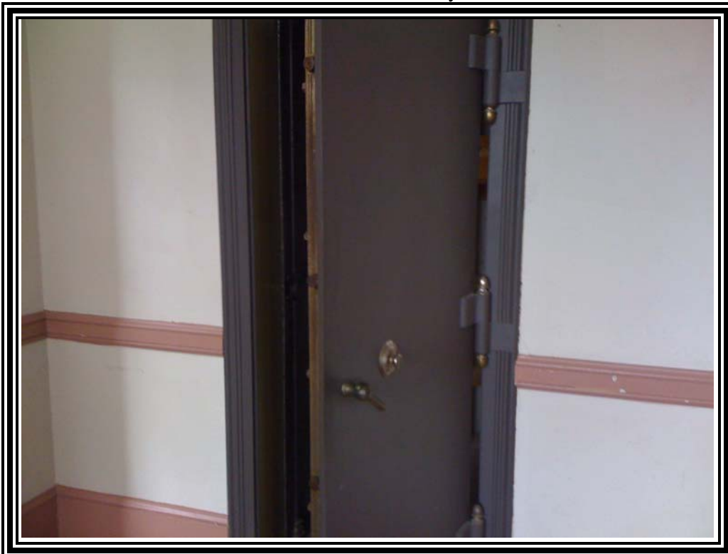
2. View of dark brown LBP on safe door and door frame, first floor Comal County Courthouse.
