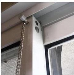
Pinning a window hut reduces the chances that the window can be pried open. This is accomplished by drilling a hole at a slightly downward angle through both the movable and fixed window frame and placing a pin, nail, or eyebolt in the hole.
